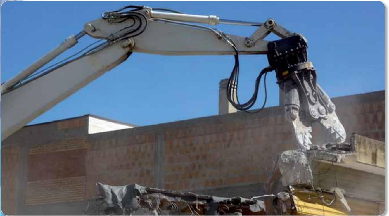
The field of **demolition** represents one of the main applications of pressure intensifiers. In this field, the weight of the cylinders linked to the demolition crusher, permits more extension of the operating machine arm they are connected to. The use of an intensifier allows reducing the cylinder diameter or employing crushers with a higher closing force.
